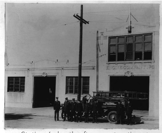
Station 6 shortly after construction Circa 1915
